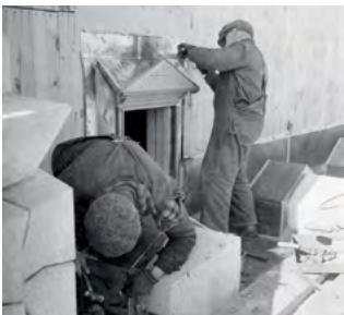
Copper is laid on one of the four turrets.
