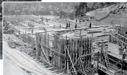
The construction site in its early stages, with no apparent structure.
