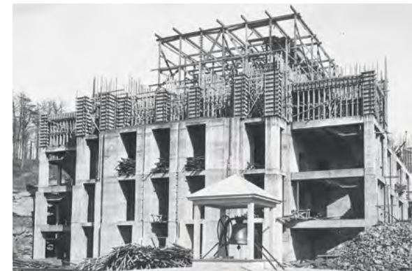
The church under construction seems firmly anchored in the mountain.
